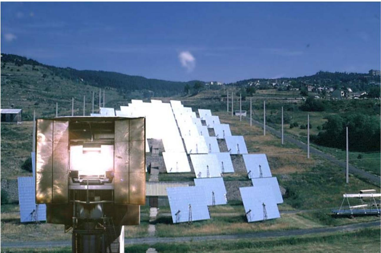
**Figure 1:** Heliostats field and focal point of the 1MW solar furnace at PROMES-CNRS in Odeillo, France
