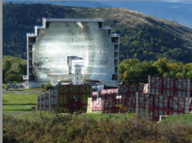
1 MW CNRS solar furnace for testing the solar pilot plant
